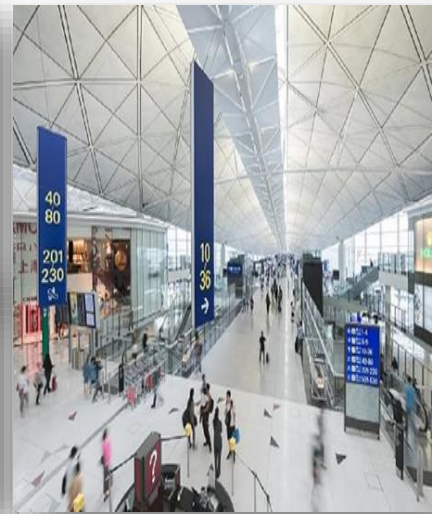
Hong Kong International Airport
