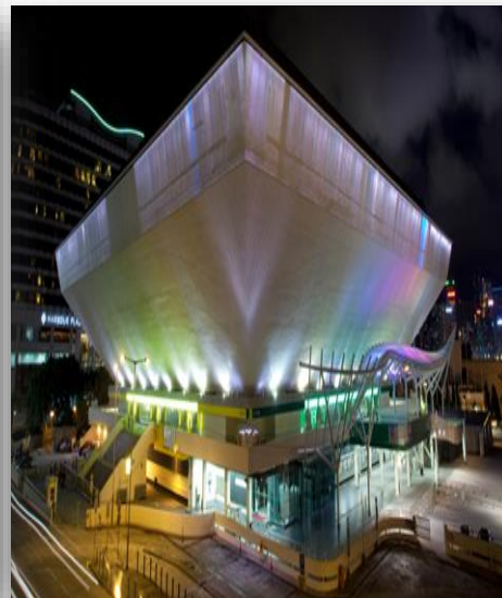
LED Display Systems at HK Coliseum – Smart Solutions
